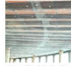
reinforcement for cooling/heating ceilings with dowels type AD
