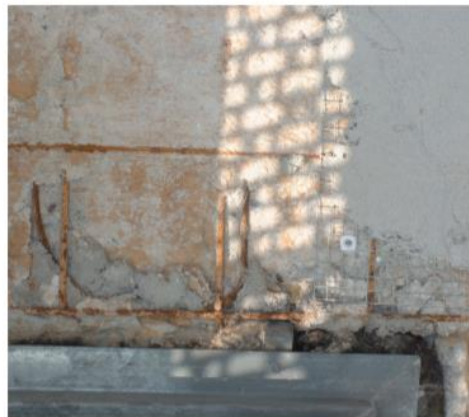
Armanet protection on bad undergrounds
